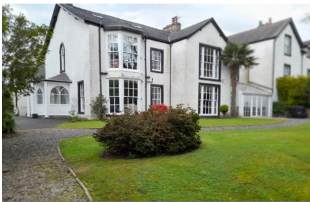
Gawithfield House - front view
