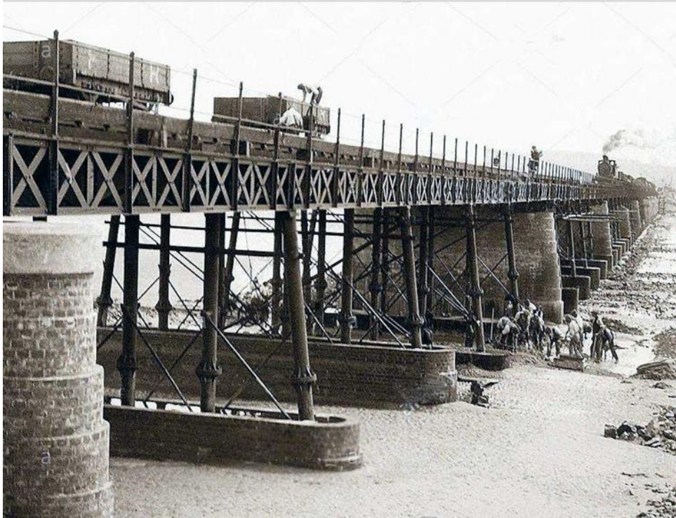
Arnside viaduct bricking same process for Leven viaduct
