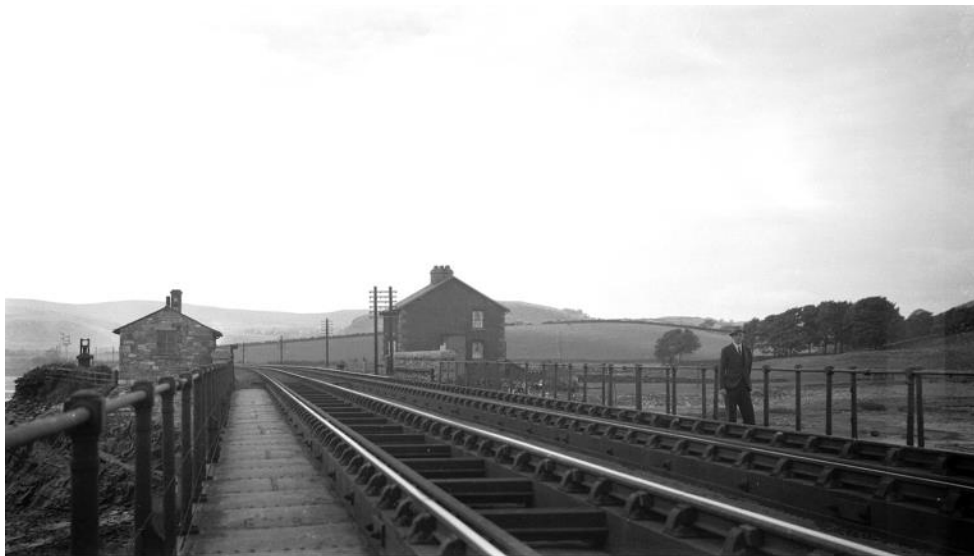
West end of viaduct showing cottages and wind speed indicator to left of cottages
