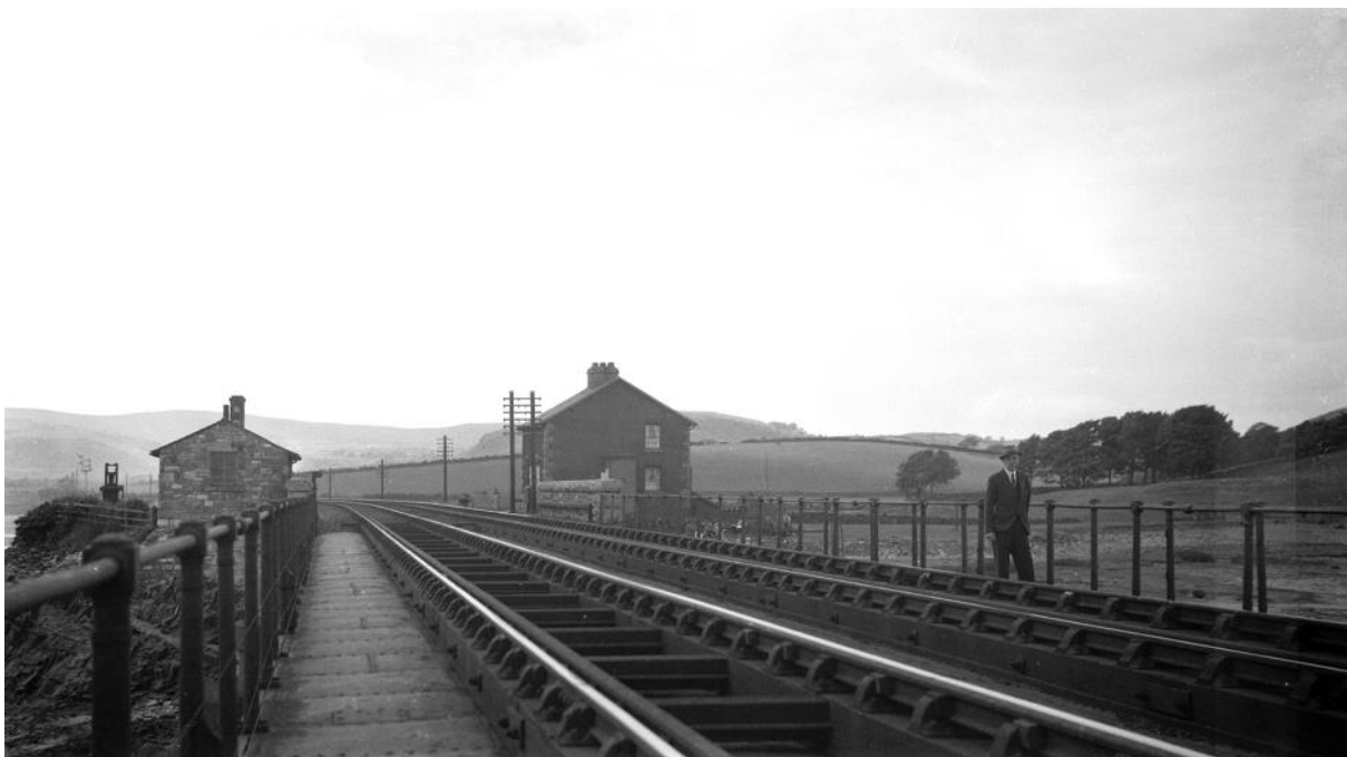
West end of viaduct showing cottages and wind speed indicator to left of cottages
