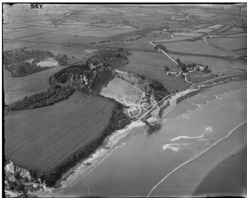
Plumpton Viaduct with the remains of Plumpton Pier in the foreground
